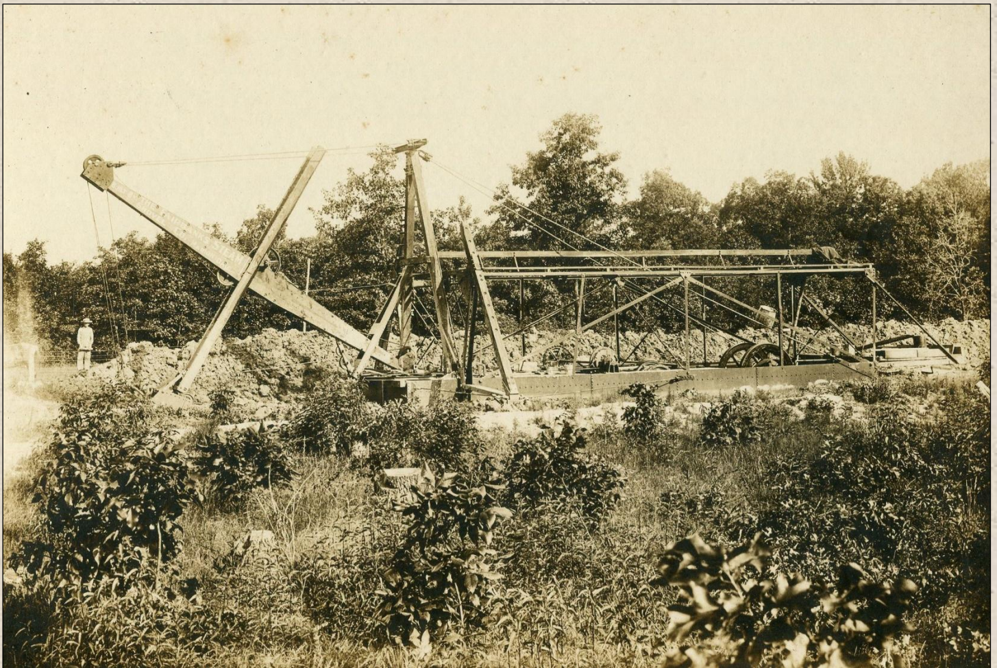
This photograph from Riceland Foods' archives is labelled "Ed McGahhey 1907 dredge boat ditch west of Stuttgart to drain city."
